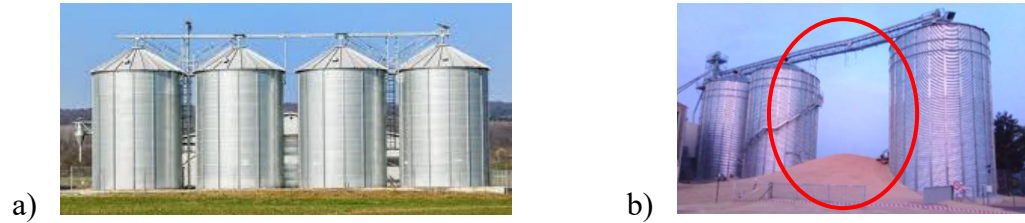
Fig. 2: Steel silos a) without failure, b) collapse of a silo for the storage of approximately 120 t of wheat
