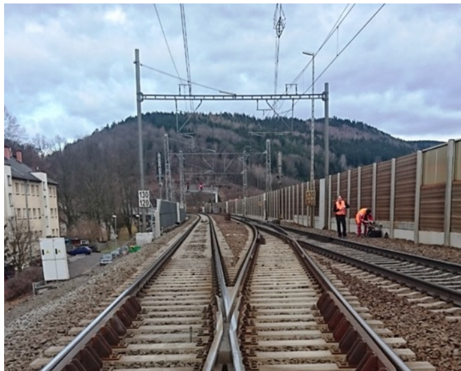
Fig. 1: View of rail coupling with switches 3 and 4.
