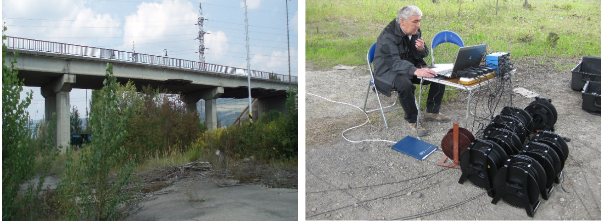
Fig. 6: View of the tested bridge and the measuring centre
