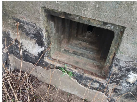
Fig. 4: Remains of the original plaster.
