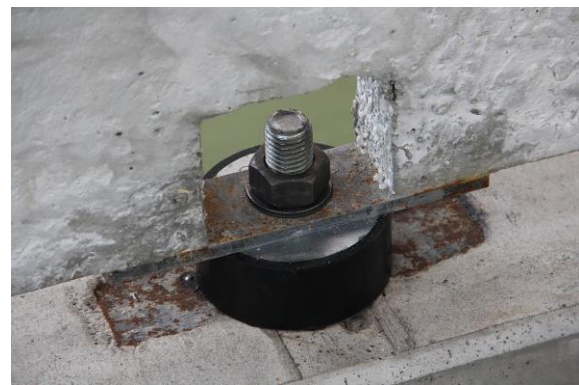
Fig. 4: Soft connection with elastomeric bearings.
