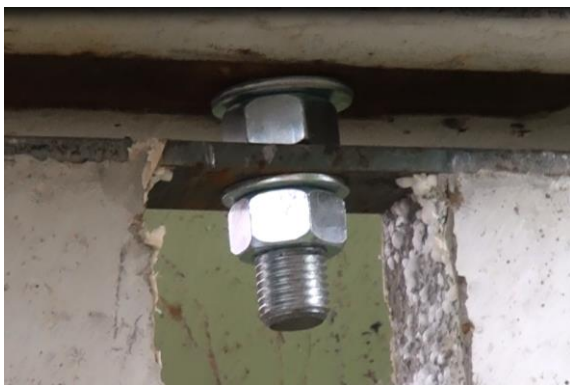
Fig. 3: Rigid connection with steel screw fasteners.
