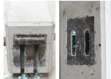
Fig. 2: Embedded steel elements.
