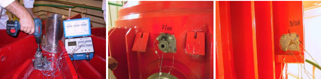
Fig. 4. View to individual measurement locations, a) drilling in location 1, b) hole-drilling equipment at location 2 after removing milling machine, c) strain-gage after drilling, location 3.
