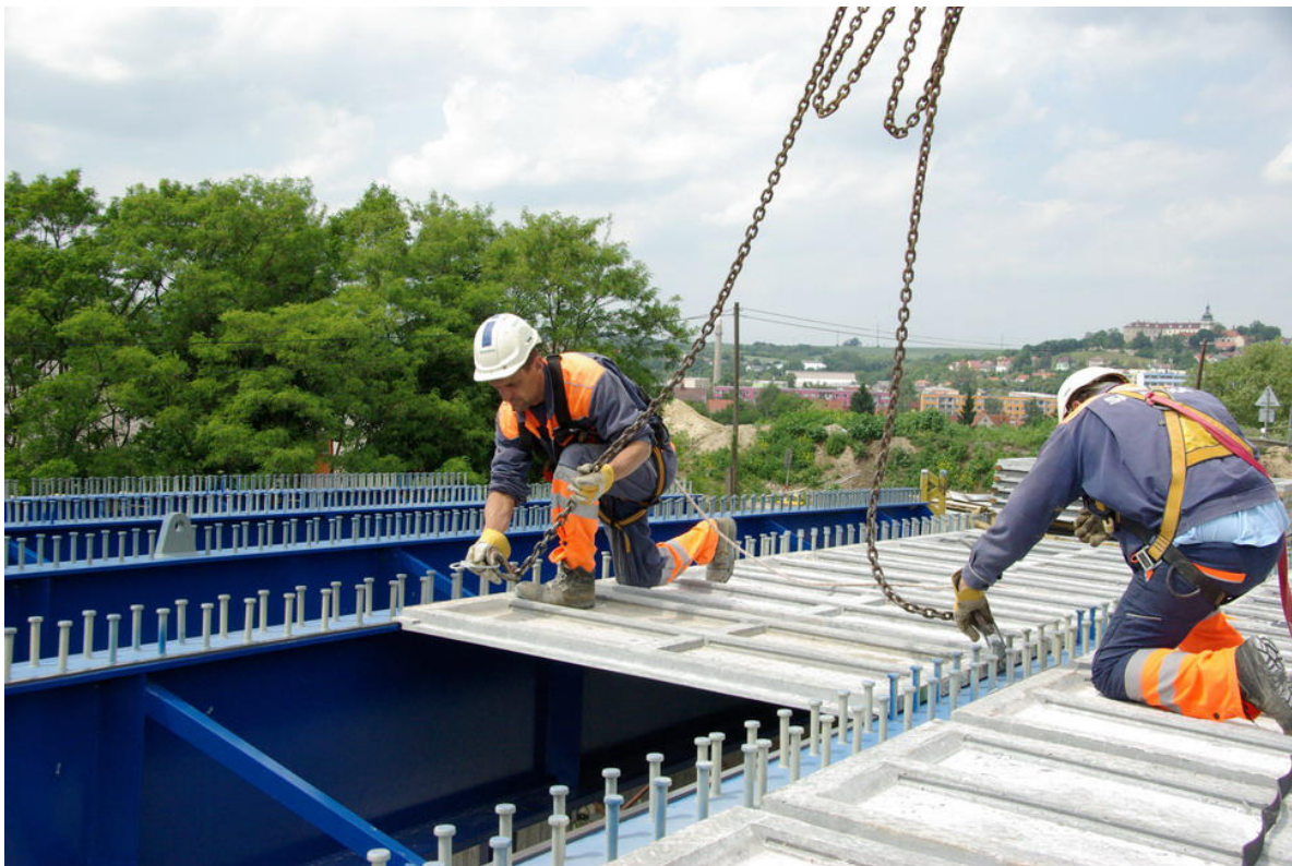
Fig. 1. Installation of lost shuttering UHPFRC slabs.
