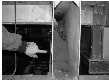
**Fig. 3.** Deformed webs of beam.
