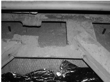
**Fig. 2.** Burned-out of framework joint sheet.
