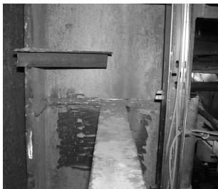
**Fig. 4.** Joining of U-profile to the column S2L.
