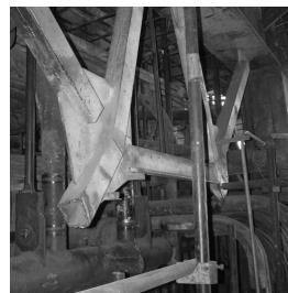
**Fig. 5.** Removed struts from left side of boiler (U-profile web is on right side).
