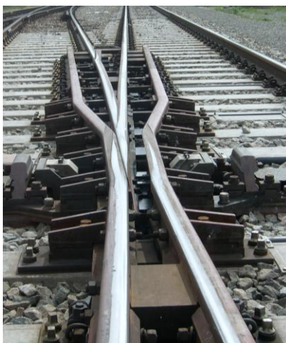
Fig. 1 Tested railway substructure with turnout
